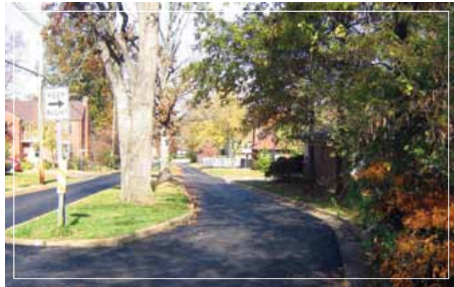
After UTBAWS application, Center Dr. between Gannon and Cornell
