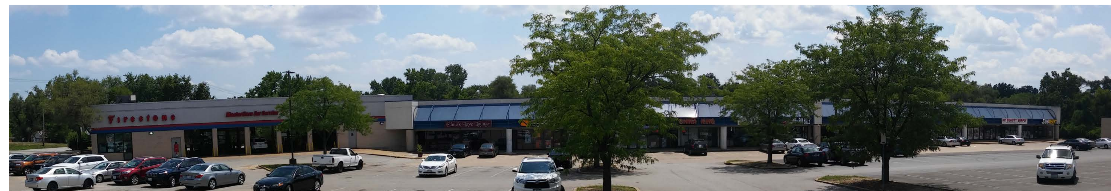
OVERALL EXISTING BUILDING PHOTO ELEVATION N.T.S.
