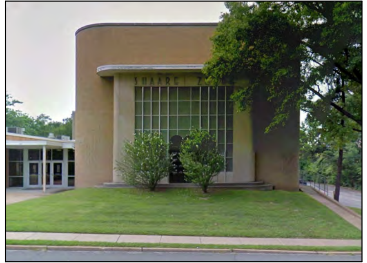
EXISTING SANCTUARY WINDOW FROM HANLEY RD.
