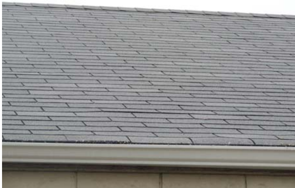
PHOTO #5: Asphalt shingle roof
