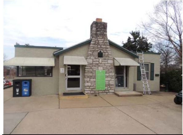
PHOTO #2: Side east elevation
