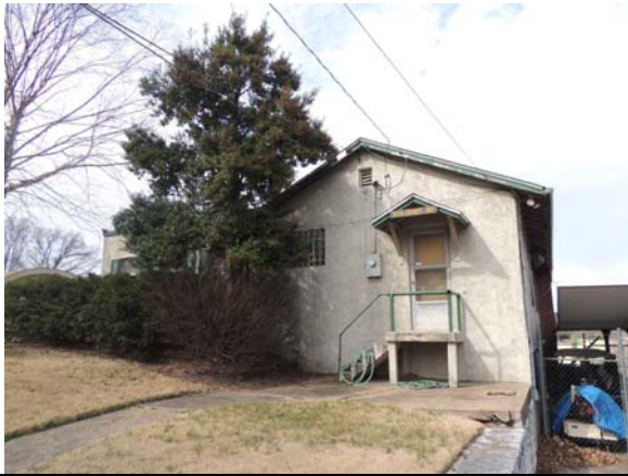
PHOTO #1: Front south elevation
