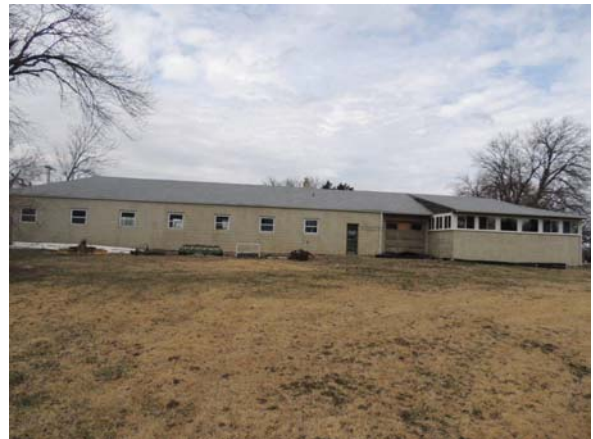
PHOTO #4: Rear south elevation
