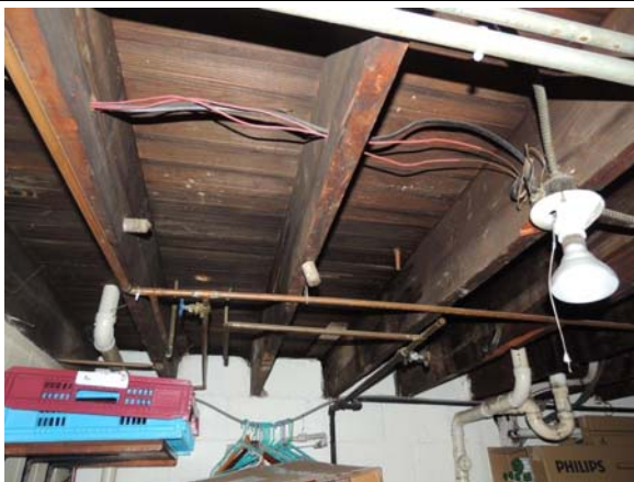
PHOTO #39: Lower level storage area
