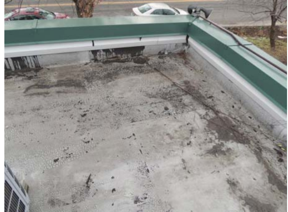
PHOTO #8: Lower roof
