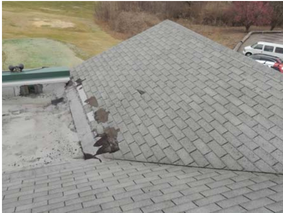
PHOTO #7: Main roof
