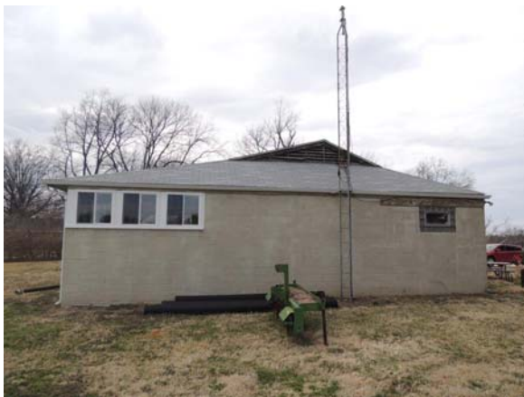
PHOTO #3: Side east elevation
