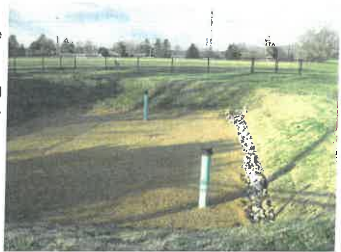
Surface Sand Filter, St. Louis County, MO
