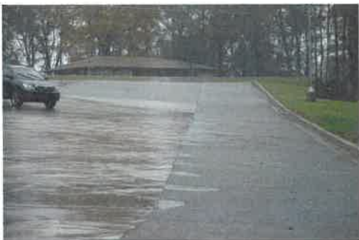
Permeable Pavement During Rainfall
