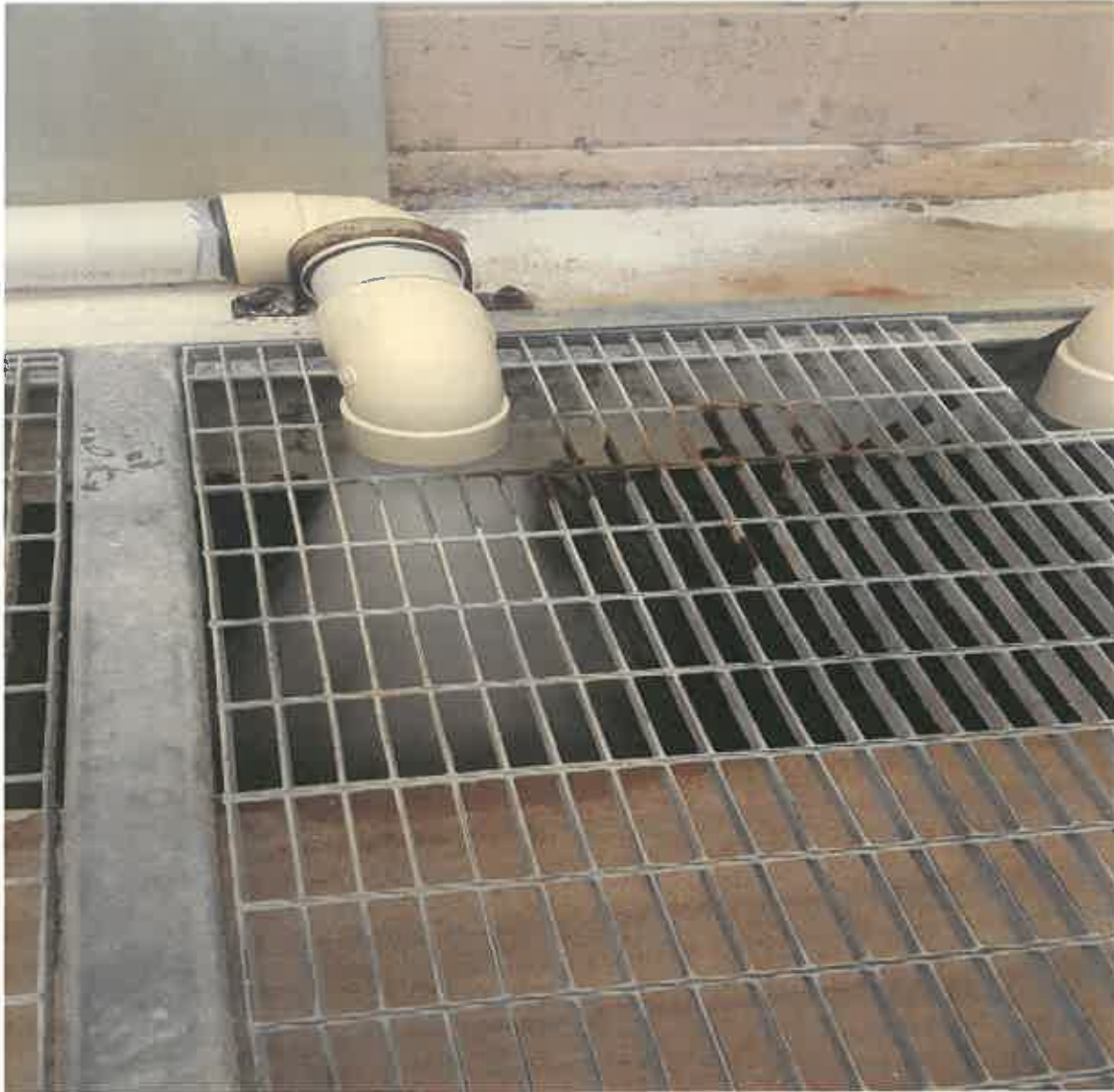
SIX INCH MAIN RE-FILLING THE POOL
