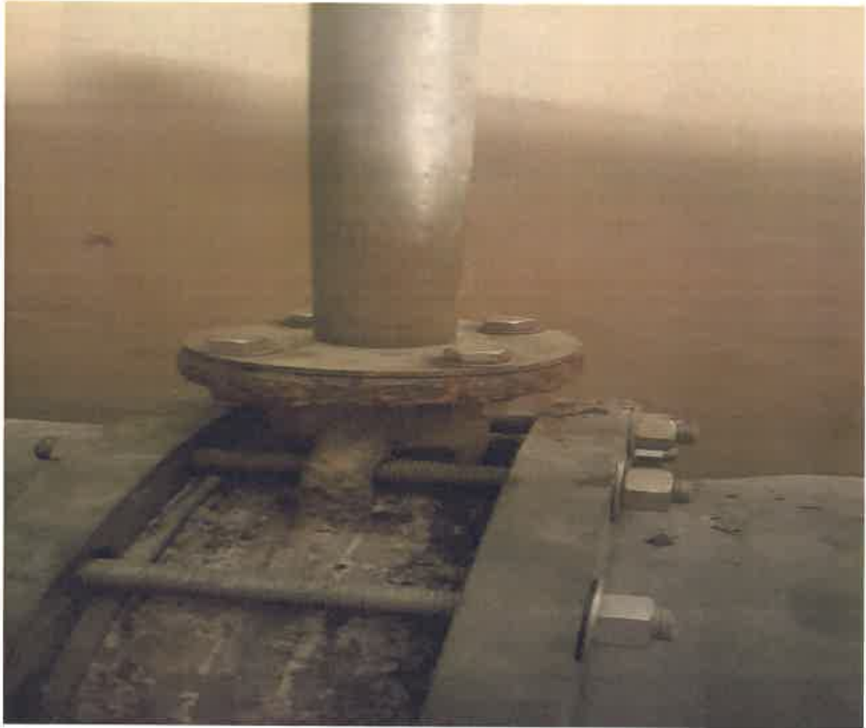
VALVE SHAFT MECHANISM IS REPAIRED
