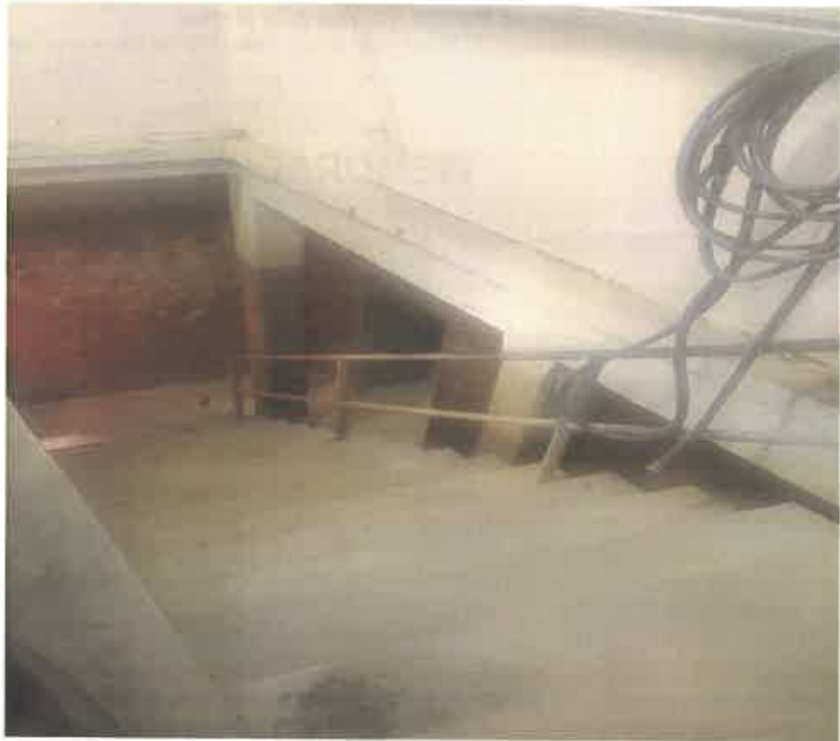
STEPS LEADING TO SLURRY PIT
