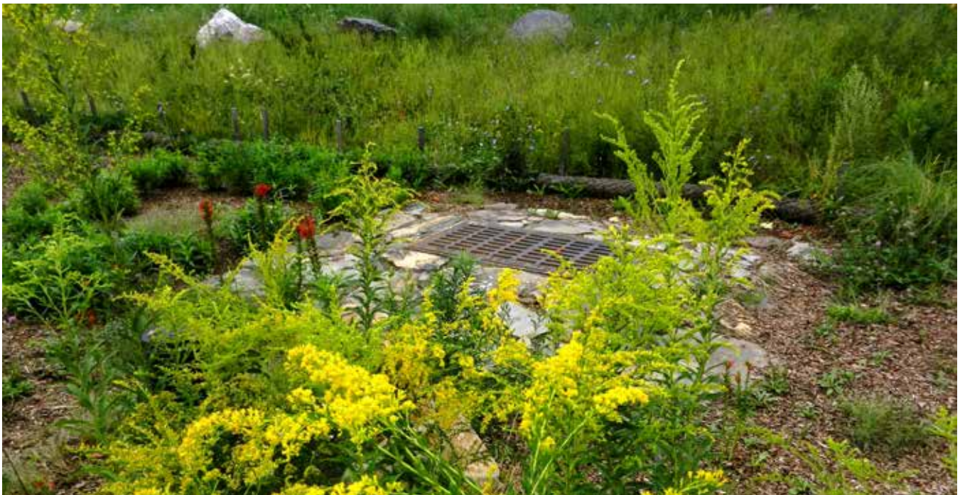
North and South Conduit BMP, New York, New York
