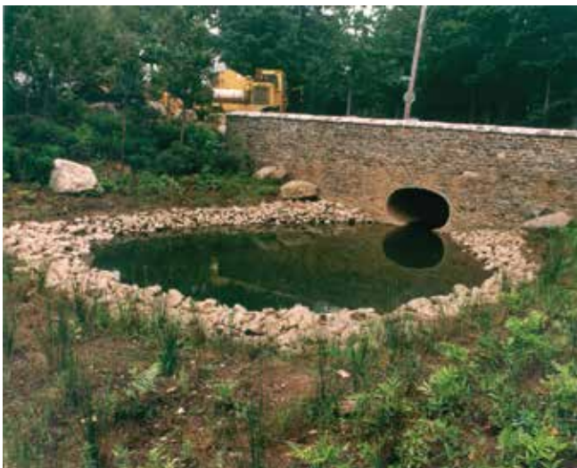
Stiling basin used in the Staten Island Bluebelt, NY to reduce sediment.
