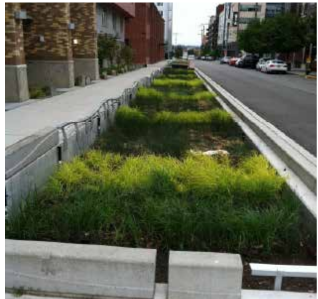
Stormwater structural control in Seattle, WA
