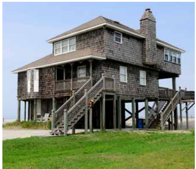
Houses meeting freeboard requirements in coastal areas by raising living spaces to the required height above the 100-year flood elevation.
