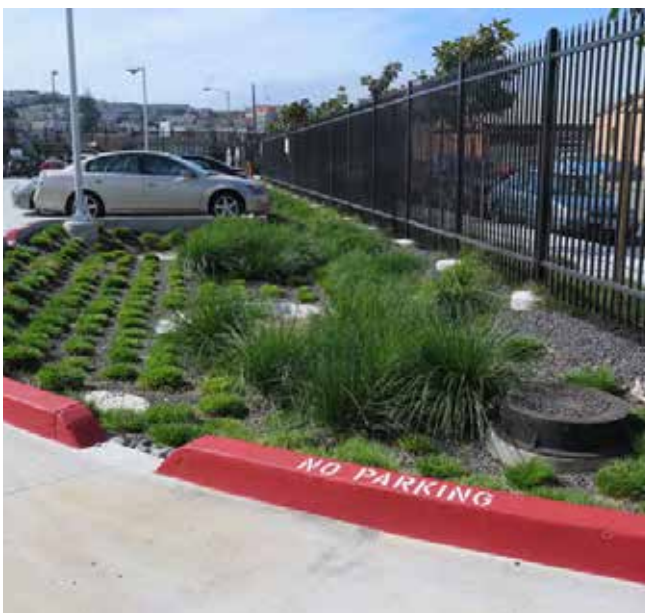
Bioretention in a parking lot of an industrial site in San Francisco, CA
