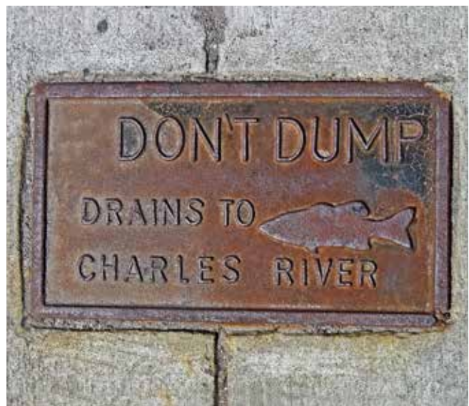
Catch Basin Casting in Boston, MA
