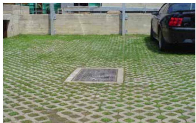
Apartment parking lot with pervious paving
