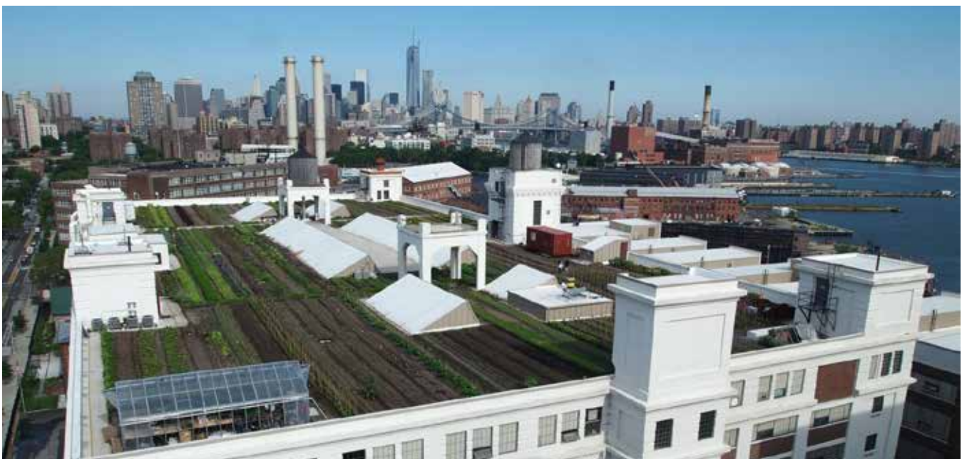
The Brooklyn Navy Yard was the recipient of a green infrastructure grant to build its green roof.
