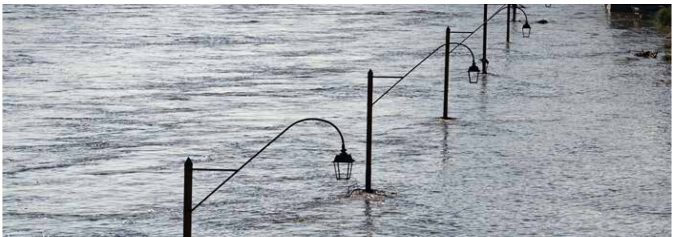
Street lamps inundated during flood; some communities choose to raise electrical infrastructure to mitigate impact during flooding events
