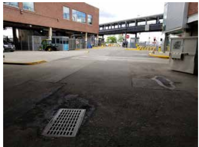
DOT yard on St. George in New York City, NY
