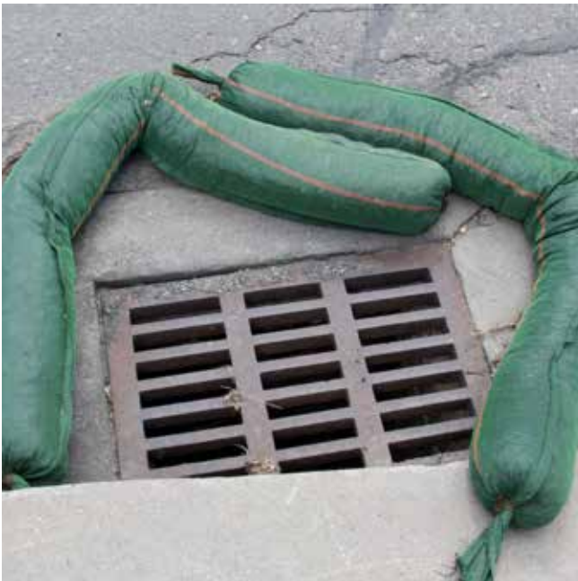
Sediment control around a storm drain
