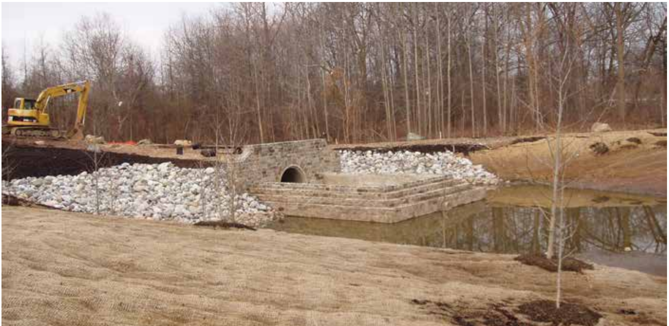
Staten Island Bluebelt in Construction in New York City
