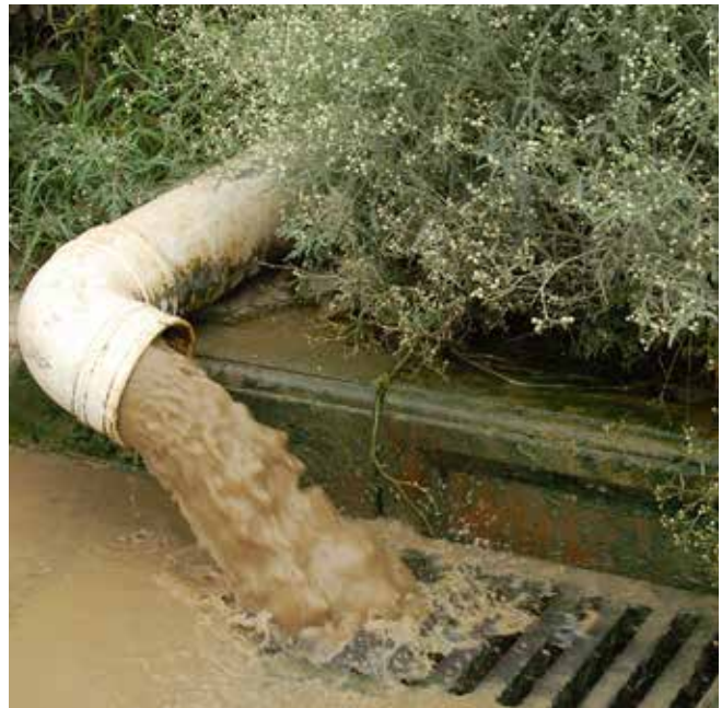
Construction runoff with sediment entering a storm drain in Arlington, VA is a hazard to the receiving streams and waterbodies.
