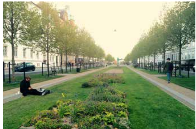
Potential site of stormwater boulevard in Copenhagen, Denmark
