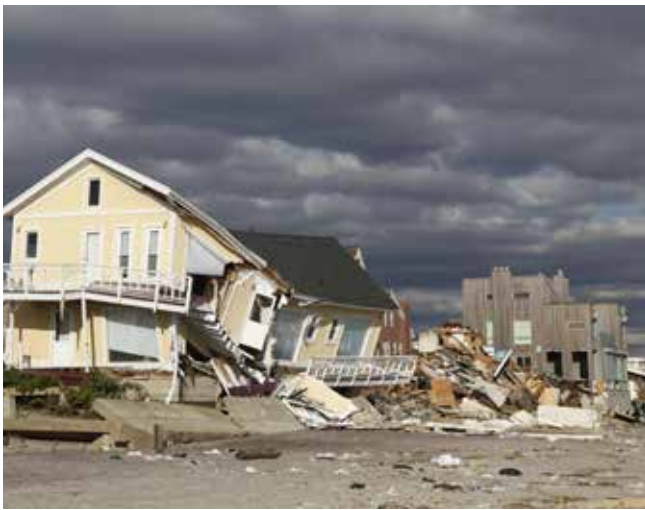
Damage from Hurricane Sandy in Far Rockaway, NY
