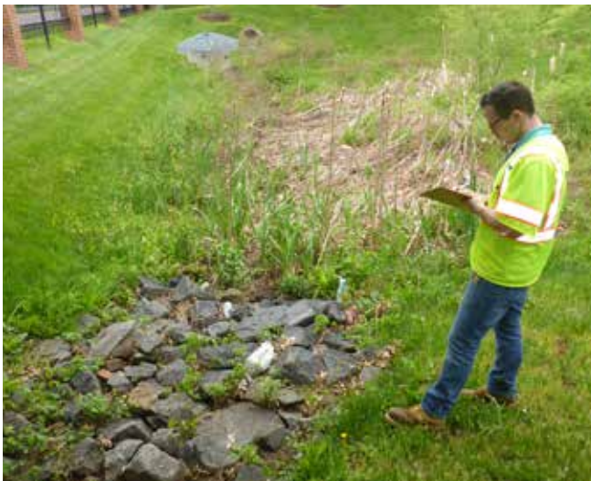
BMP inspection in Fairfax County, VA
