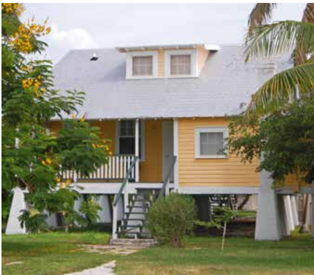
Houses meeting freeboard requirements in coastal areas by raising living spaces to the required height above the 100-year flood elevation.
