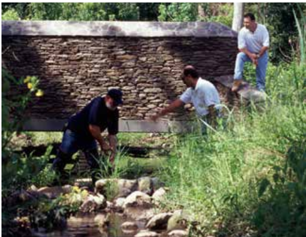
Natural habitat creation around structural stormwater controls.
