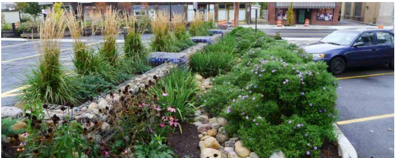
Post-construction bioretention implemented on private property in the Northeast Ohio Regional Sewer District, OH
