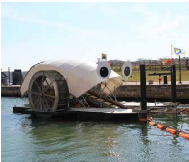
Trash removing water wheel in the Baltimore Harbor
