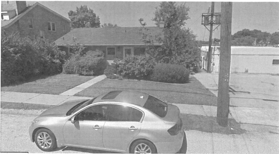
Image I. Street view of 1167 Remley Ct.
