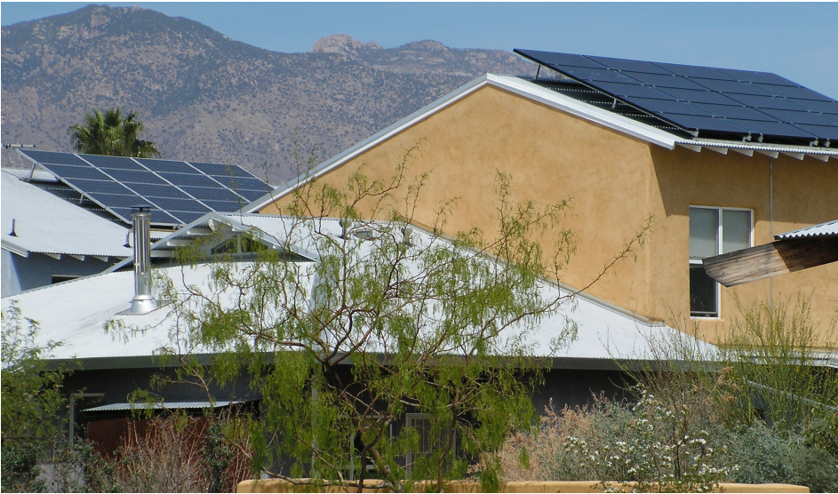
Solar panels atop homes in Tucson
