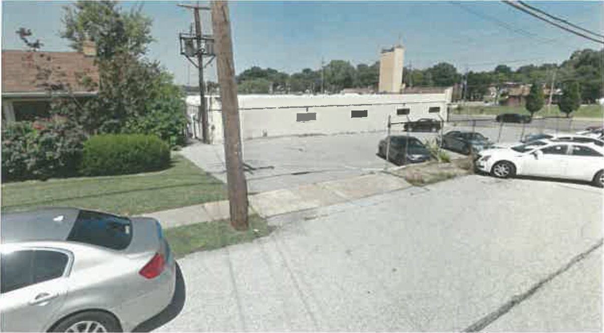
Image III. Street view of adjacent property to the North (7700 Olive)
