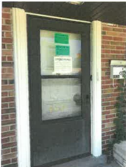
Above: A closer view of the condemnation order posted on a residence.
