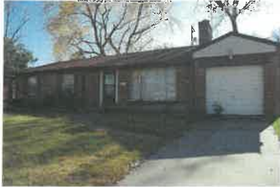
A single-family home that exhibits deterioration. This home has been condemned.
