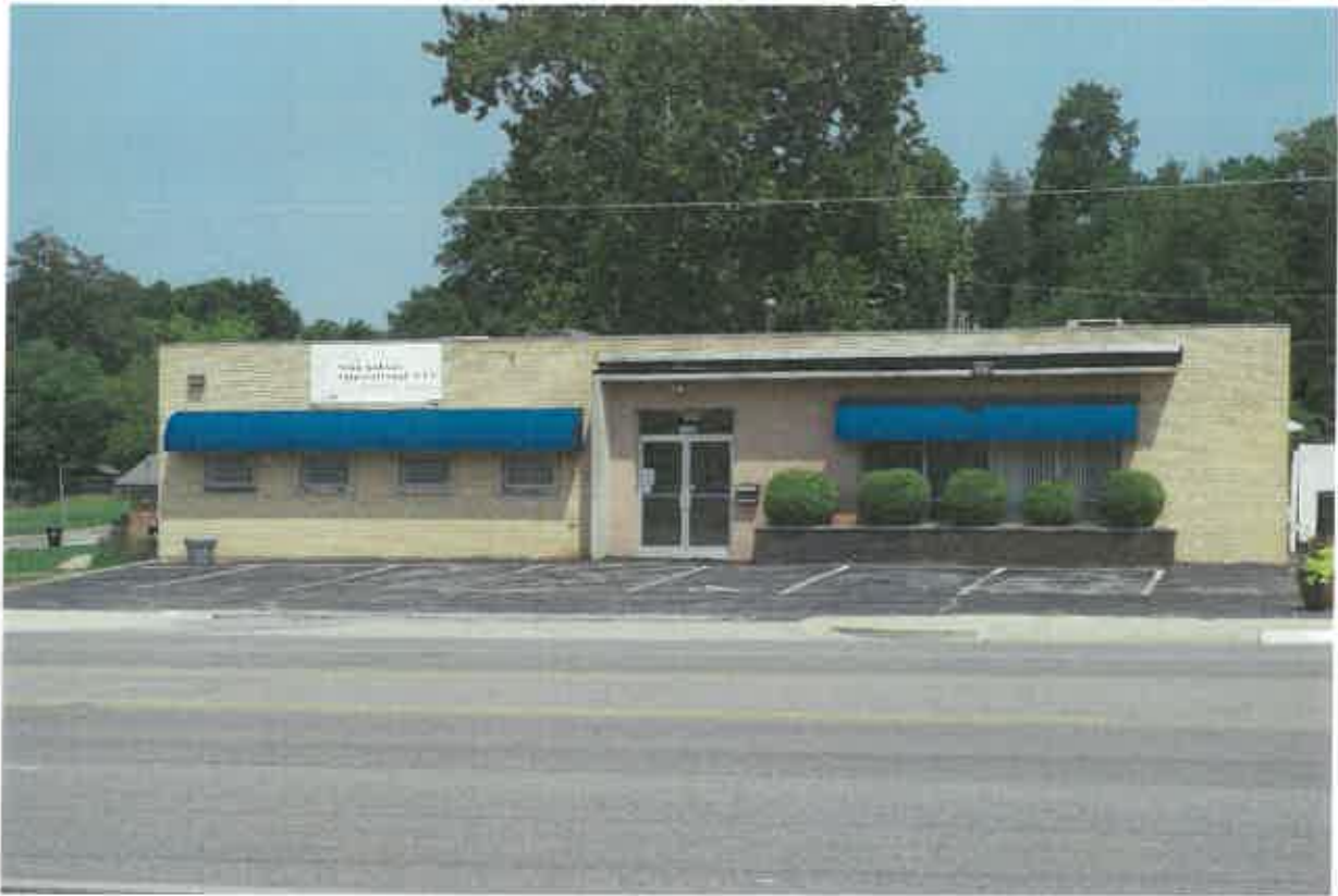
A vacant, deteriorated commercial structure.
