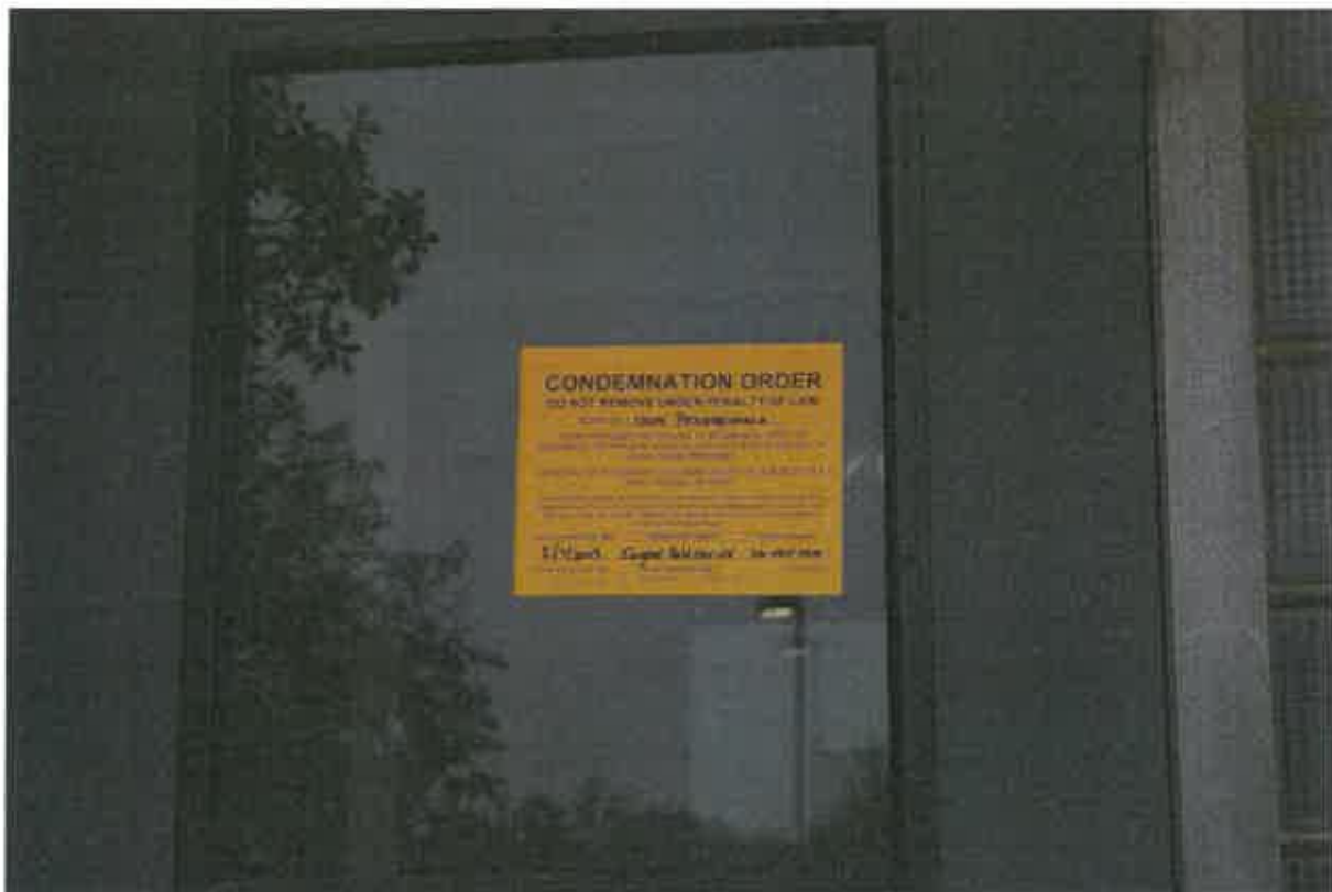
A closer view of the condemnation order posted on the building pictured above.
