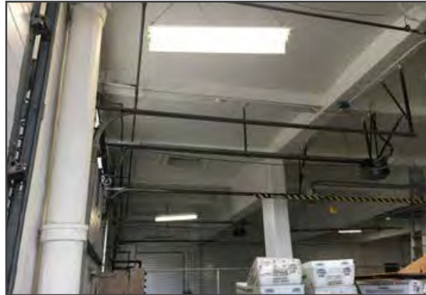
03.00 CONCRETE Board Formed Barrel Vault
