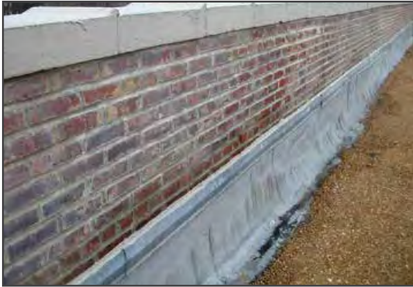
04.03 POINTING AT PARAPET
