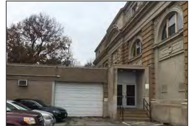
08.17 OVERHEAD DOOR Historically Inaccurate
