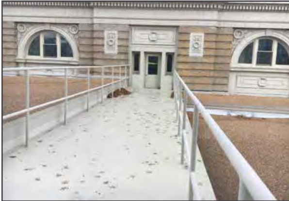
03.02 CAST IN PLACE CONCRETE SIDEWALKS & TERRACES Rooftop walk
