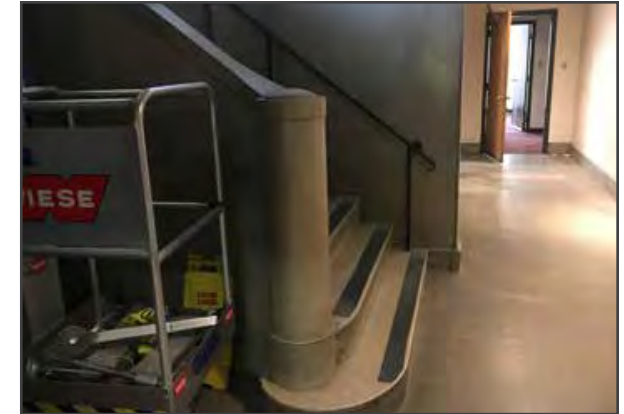
04.01 INTERIOR MASONRY CLEANING Stone Railings/Wainscoting
