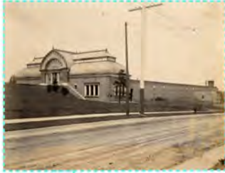
1903: ORIGINAL WOMEN'S MAGAZINE BUILDING & PRESS ANNEX BUILT
