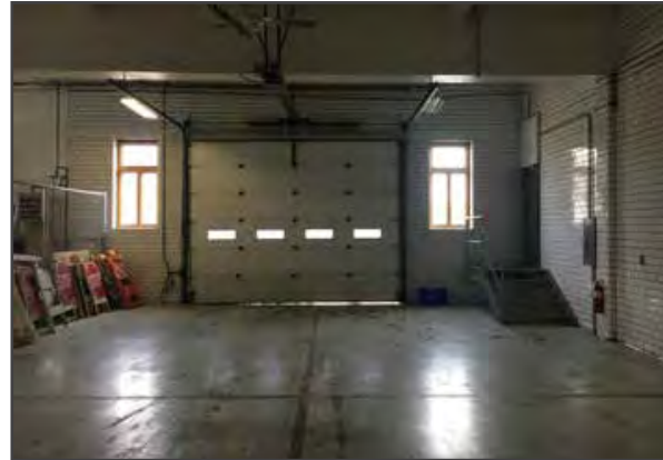
03.02 CAST IN PLACE CONCRETE Hi-bay slab
