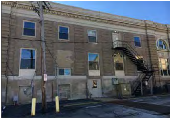
08.16 WALL VENTS Inconsistent Size and Finish
