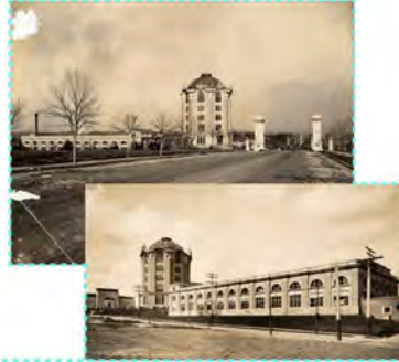
1910: COMPLETION OF NEW PRESS ANNEX (TOTAL OF 13 BAYS DESIGNED TO BETTER MATCH MAIN BUILDING)
