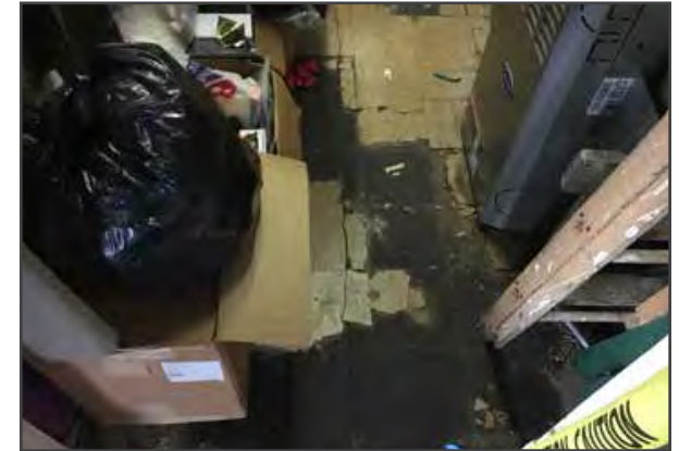
09.08 RESILIENT FLOORING Multiple Plys
