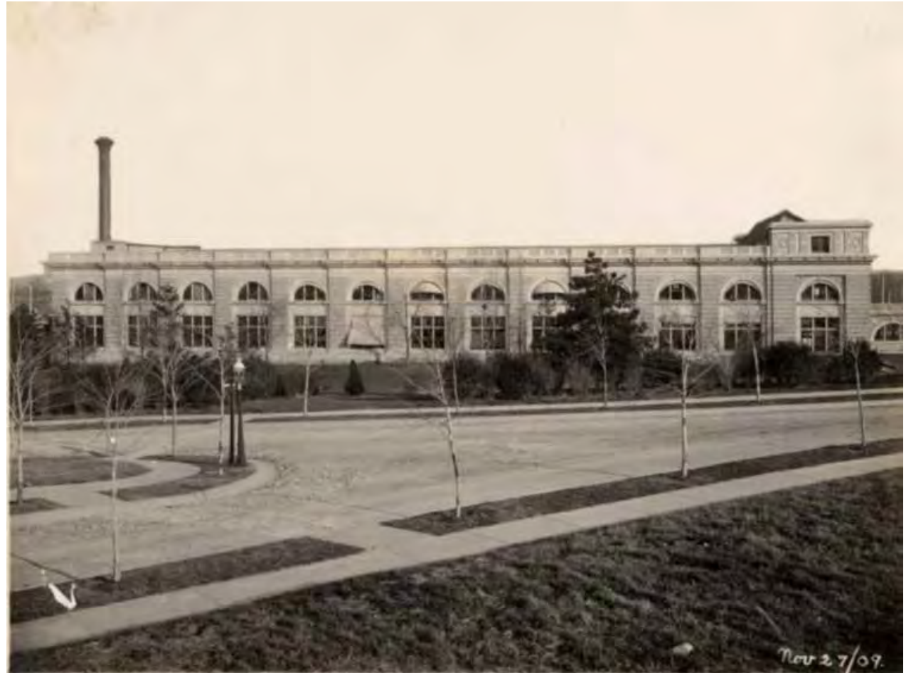
COMPLETED PRESS ANNEX: EXTERIOR
