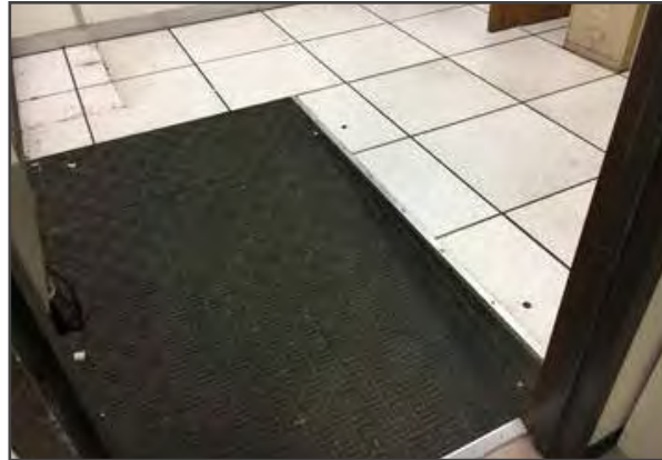
09.14 RAISED FLOOR General Condition
