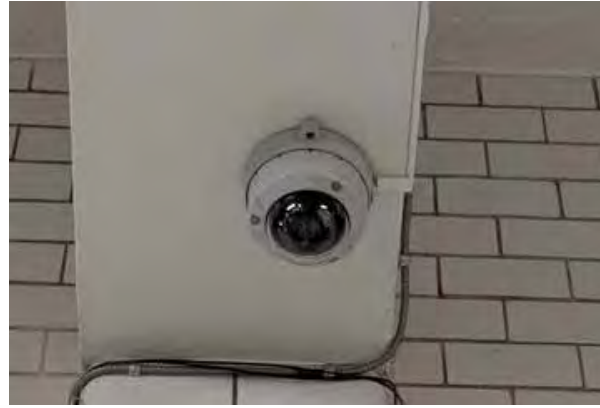
28.02 ELECTRONIC SAFETY & SECURITY Access Controls
