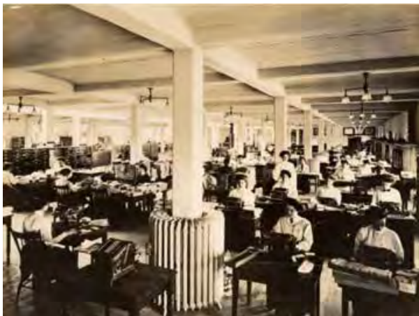
COMPLETED PRESS ANNEX: INTERIOR
