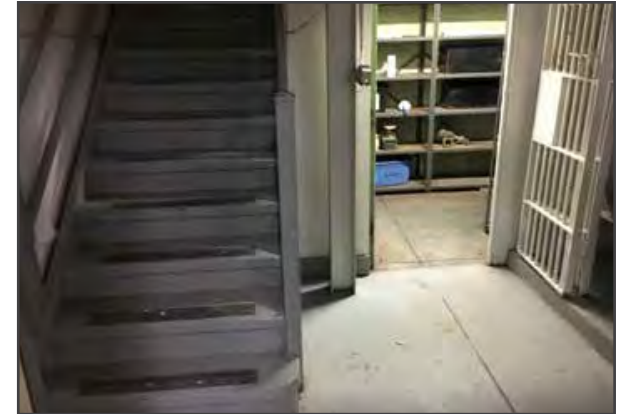
03.00 CONCRETE Exposed Slab on Grade
