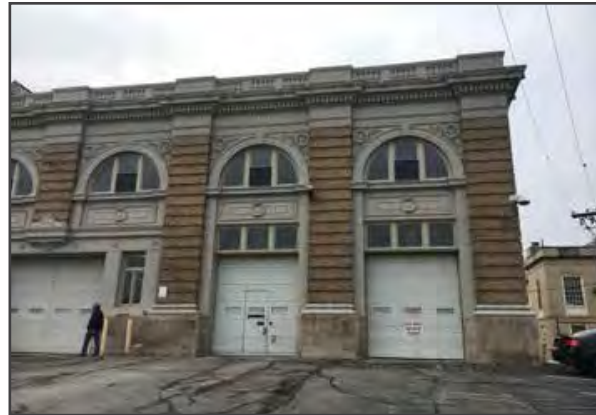
08.17 OVERHEAD DOOR Historically Inaccurate
