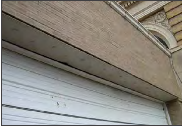
05.12 STEEL LINTEL AT GARAGE DOOR
