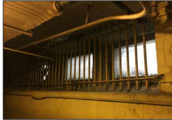
05.03 DECORATIVE METAL RAILINGS Window Security Grille
