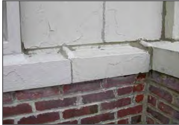
04.03 POINTING AT THIRD FLOOR CORNICE
