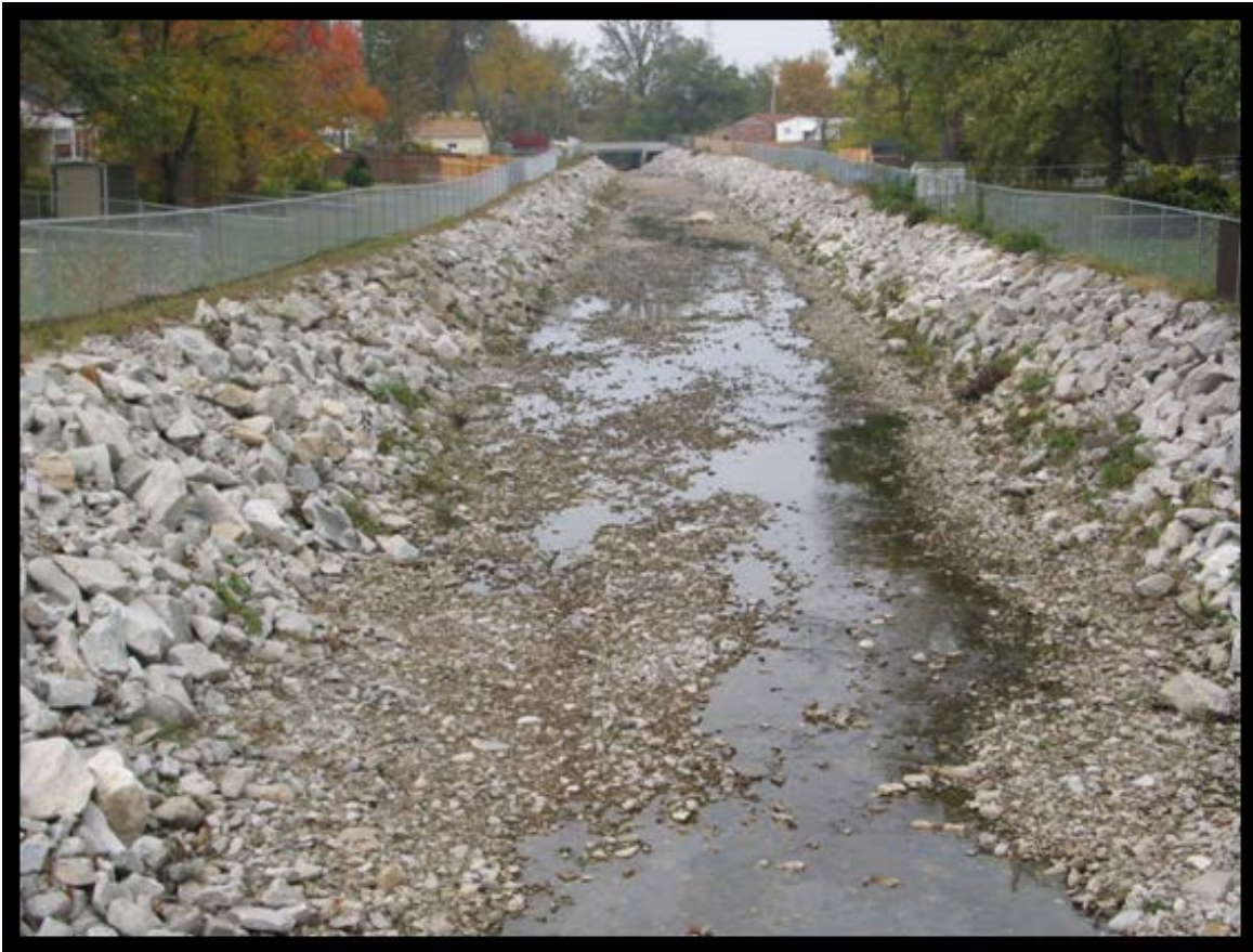
Figure 4 – Picture of Channel Improvements between RM 2.828 and RM 3.485
