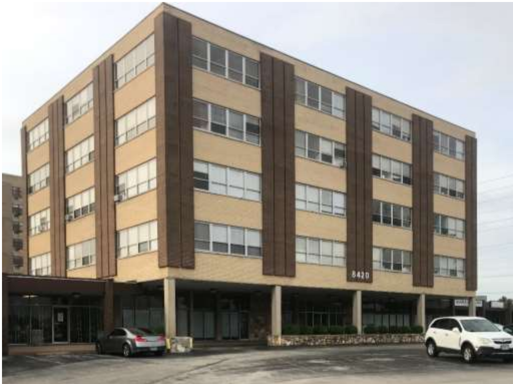
8420 Building with window AC units
