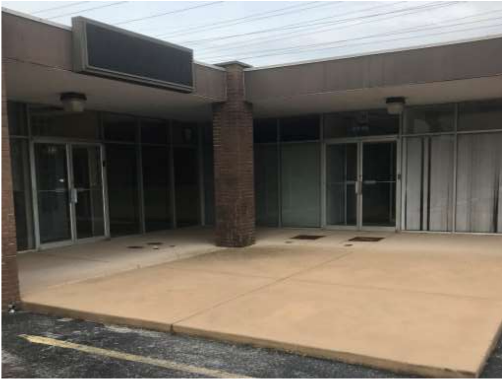
Vacant ground level retail spaces
