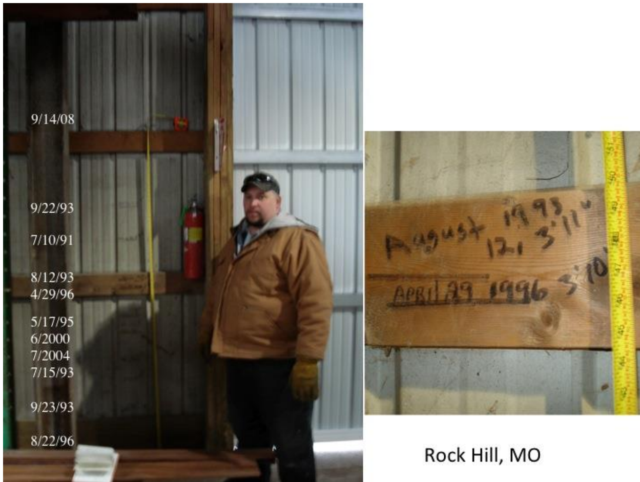
Figure 3. Left. Examples of Flood Marks scribed on the wall of a warehouse in the Deer Creek floodplain, Rock Hill, St. Louis County, MO. White lettering was added to highlight the levels and dates written on the wall. This photograph was taken in 2008, and numerous floods have occurred along Deer Creek since then. Floods prior to this record may have overtopped the Sept. 14, 2008 level. Damaging floods frequently occur on small creeks in St. Louis County. Right: Detail showing two marks located on the horizontal board to the left of the fire extinguisher. Photos by Criss.
