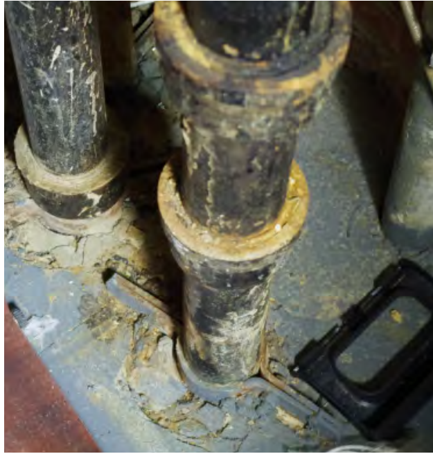
Deteriorated sewer pipes leach liquid and disintegrating particles into utility areas
