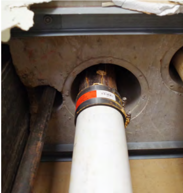
Repaired sewer pipe joined to deteriorating cast iron pipe extending between floors. Repairs to pipes between floors are considerably more difficult than those accessed behind walls.
