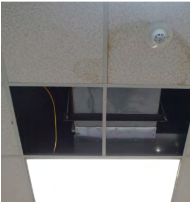
Site where ceiling tiles have been removed to determine source of leak that has damaged ceiling tiles.
