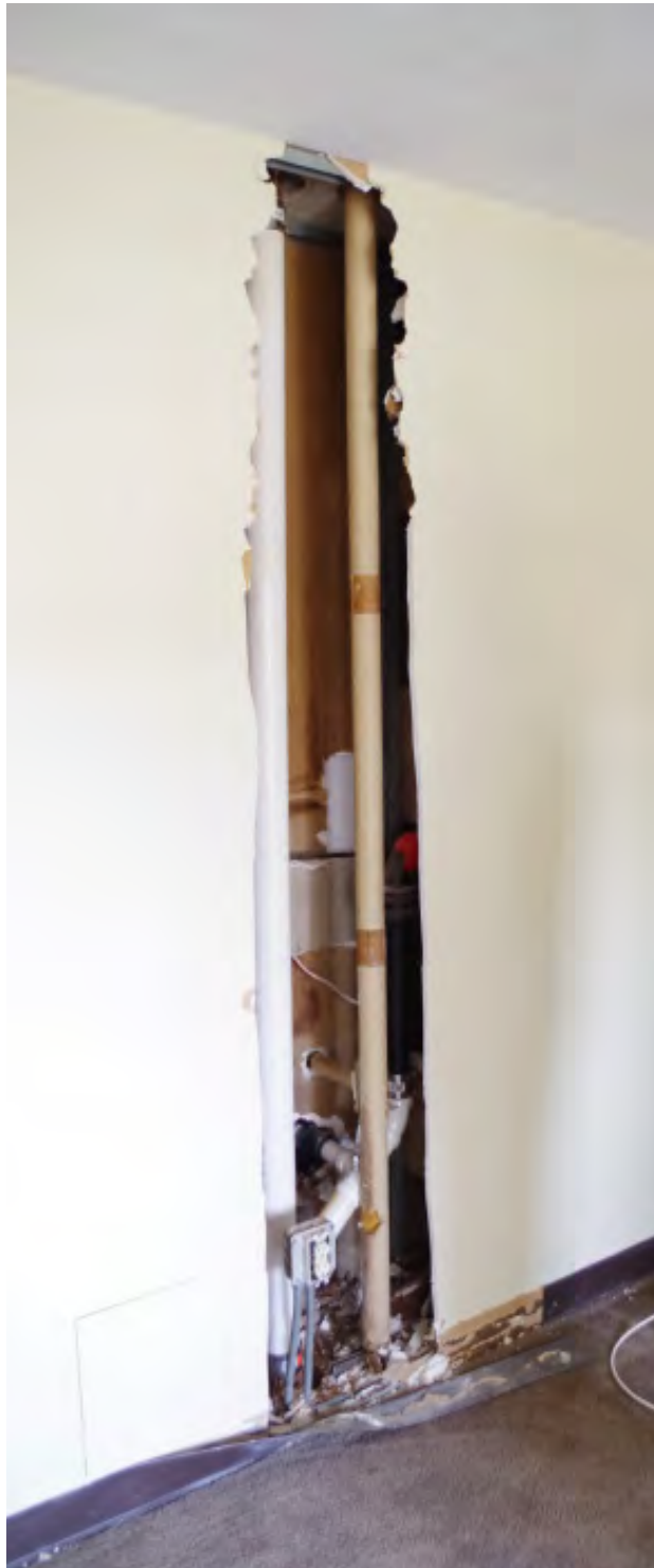
Repair in progress in apartment unit, showing floor-to-ceiling cutaway to replace corroded cast iron sewer pipe with PVC pipe
