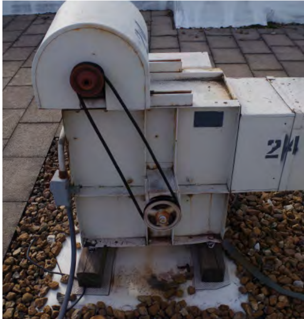
Kitchen and bath exhaust fans with exposed belts are susceptible to breakage and need replacement.
