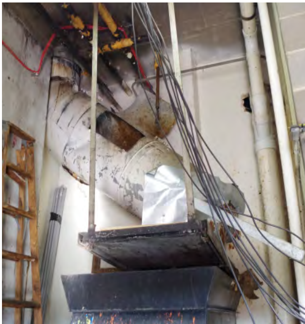
The trash chute serving the building is deteriorating and nearing the end of its useful life.
