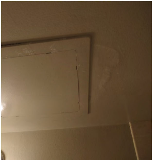
Signs of water entry and damage in an apartment unit undergoing repairs.
