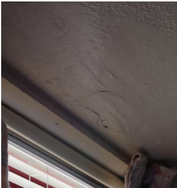
Signs of moisture entry above a window in an eighth-floor unit.
