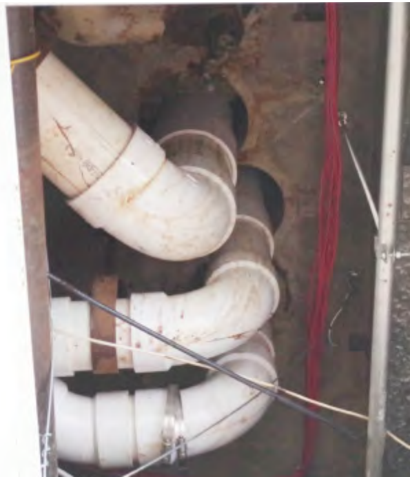
Site of pipe replacement extending into ceiling, showing discoloration to concrete structure from failing cast iron pipe.
