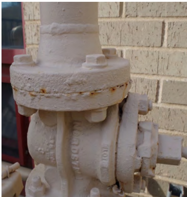
Exterior cast-iron pipes continue to rust even with regular application of paint.
