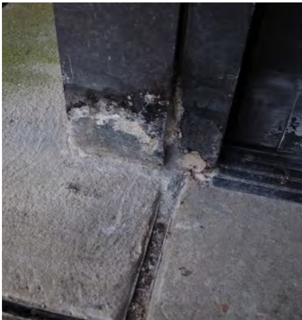
Deteriorating aluminum around main entry door.
