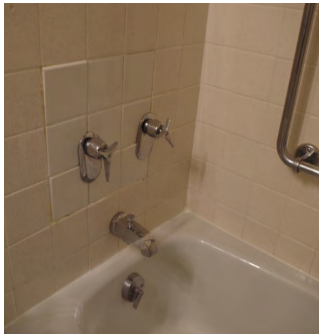
Cast-iron tubs are difficult for senior residents to use. Past plumbing repairs are evident around the faucets.
