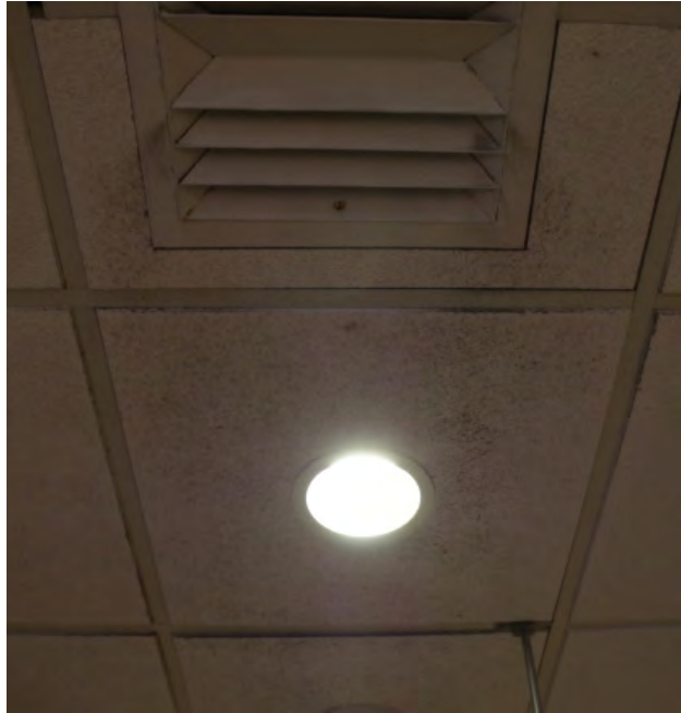
Damaged ceiling tiles from ongoing leaks in ductwork.
