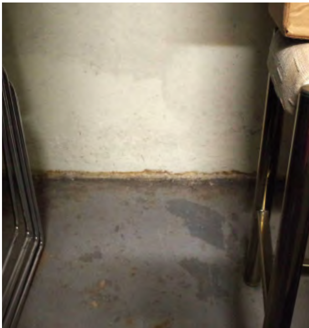
Signs of water entry within building wall and resulting damage in first floor stairwell.
