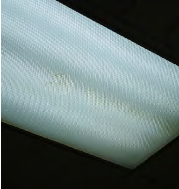
Water entry into light fixture in first floor restroom from recently-detected leak.
