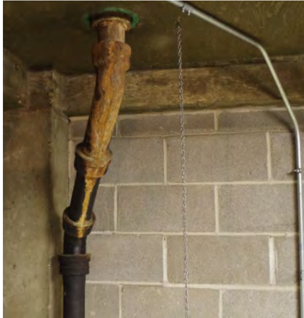
Corroding and deteriorating pipe in elevator penthouse.
