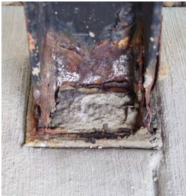
Oxidizing iron on awning posts near main entry door.
