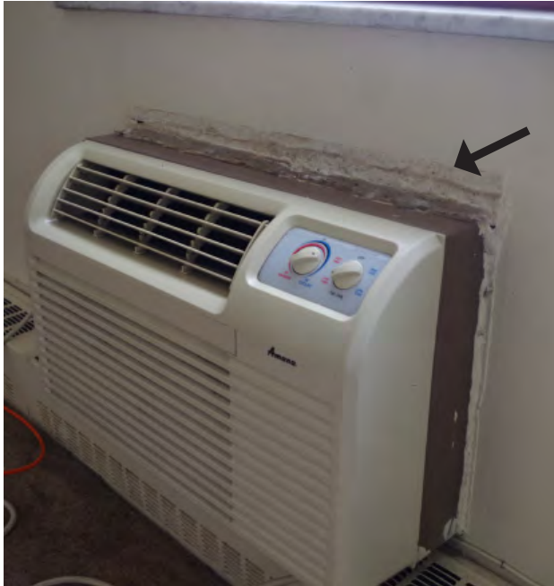
Through-wall PTAC units throughout the building require ongoing maintenance to avoid energy loss and moisture damage when seals fail.
