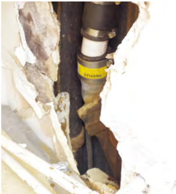
Recently repaired sewer pipe in eighth floor apartment whose failure led to water damage in the unit below.
