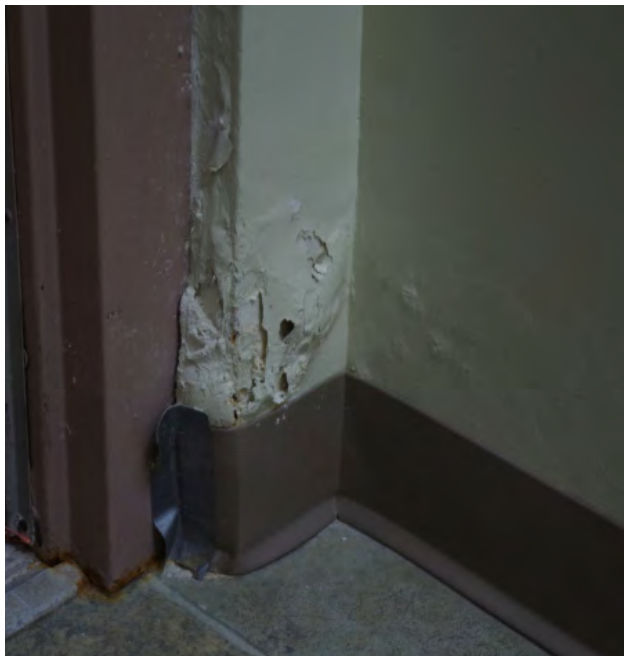
Water entry damage around exterior door, first floor.
