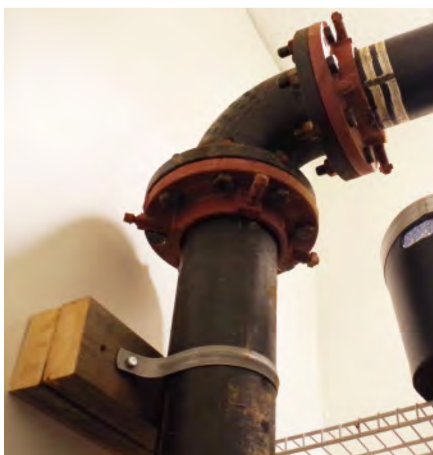
Oxidation on the exterior of a fire sprinkler riser
