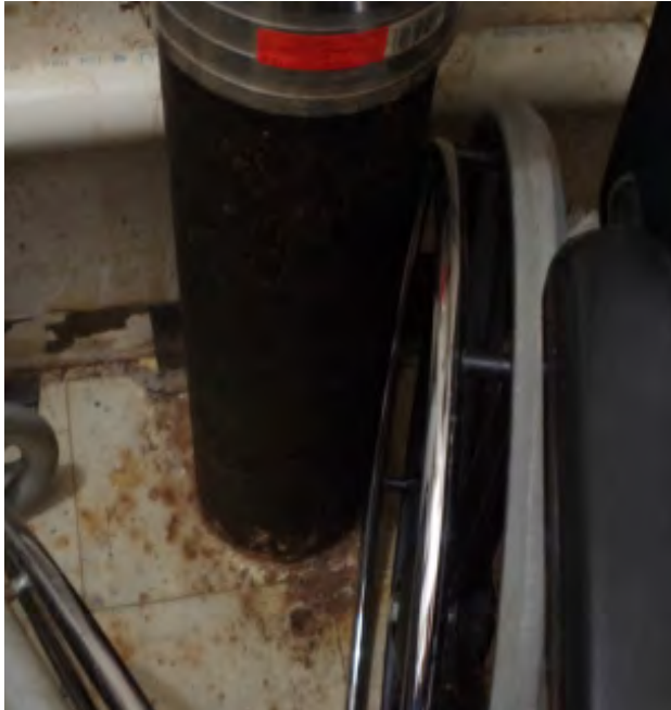
Discoloration of floor tiles as a result of oxidizing pipes
