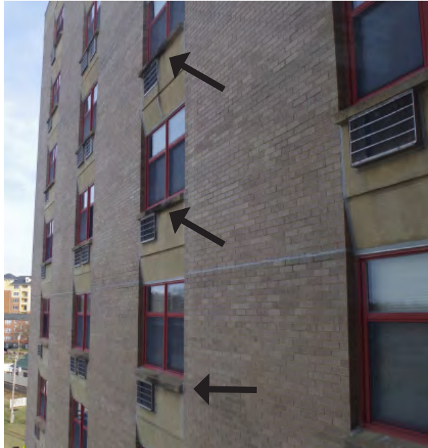
Condensation from through-wall PTAC units causes moisture to accumulate on the building exterior and discoloration and deterioration of the surrounding areas.
