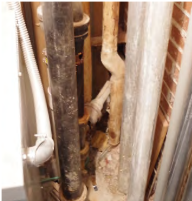
Damaged and corroding pipes
