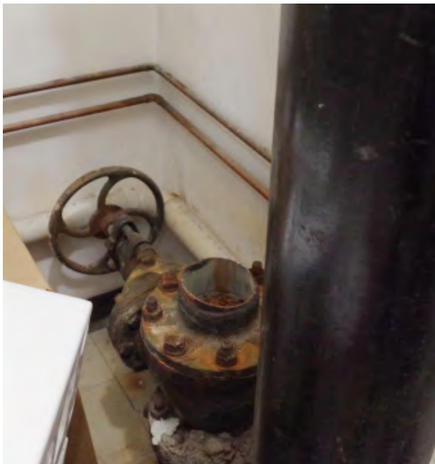
Oxidizing iron fire sprinkler riser
