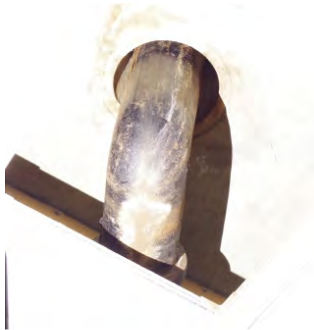
Cast iron sewer pipe extending into ceiling, showing signs of corrosion and oxidation, as well as damage to the surrounding wall.
