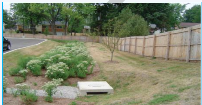
Rain gardens near sewers are one example of a BMP used to minimize strain on stormwater systems
