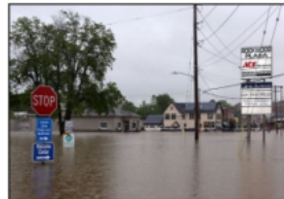
Eureka downtown area impacted by Meramec River flooding for the second time in 16 months.
