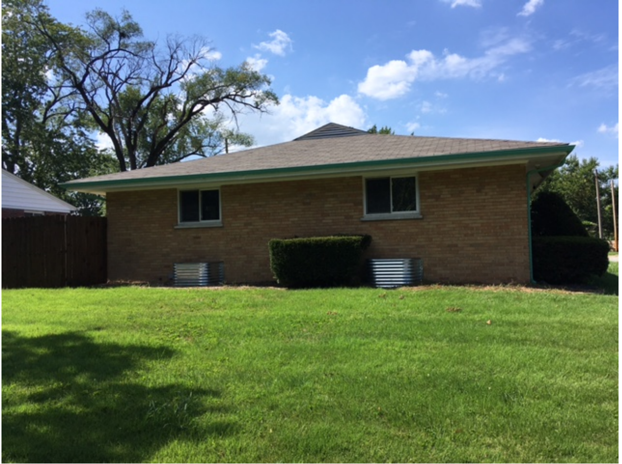
1035 Groby Rd – Note metal window barriers, open on top to admit light
