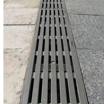
Trench Drains ( cast iron )
