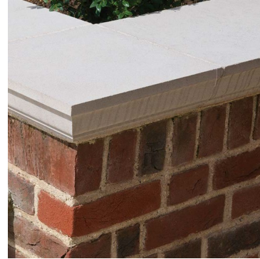
Seatwall ( brick + precast cap )
