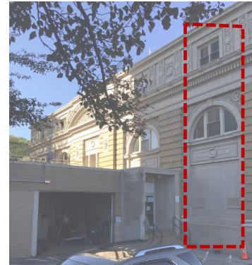
partial south facade
