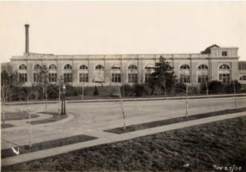
1940: fire at annex building left only 5 original bays remaining
