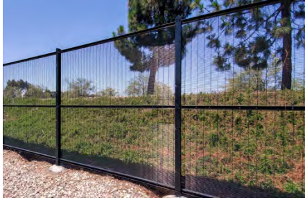
Security Fence 8' tall, anti-climb
