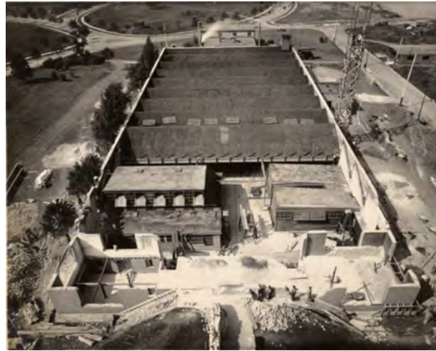
1908: deconstruction & reconstruction of press annex
