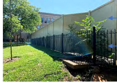
Ornamental Fence (existing)
