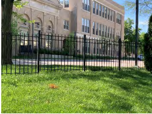
Existing ornamental fence at the Lewis Collaborative
