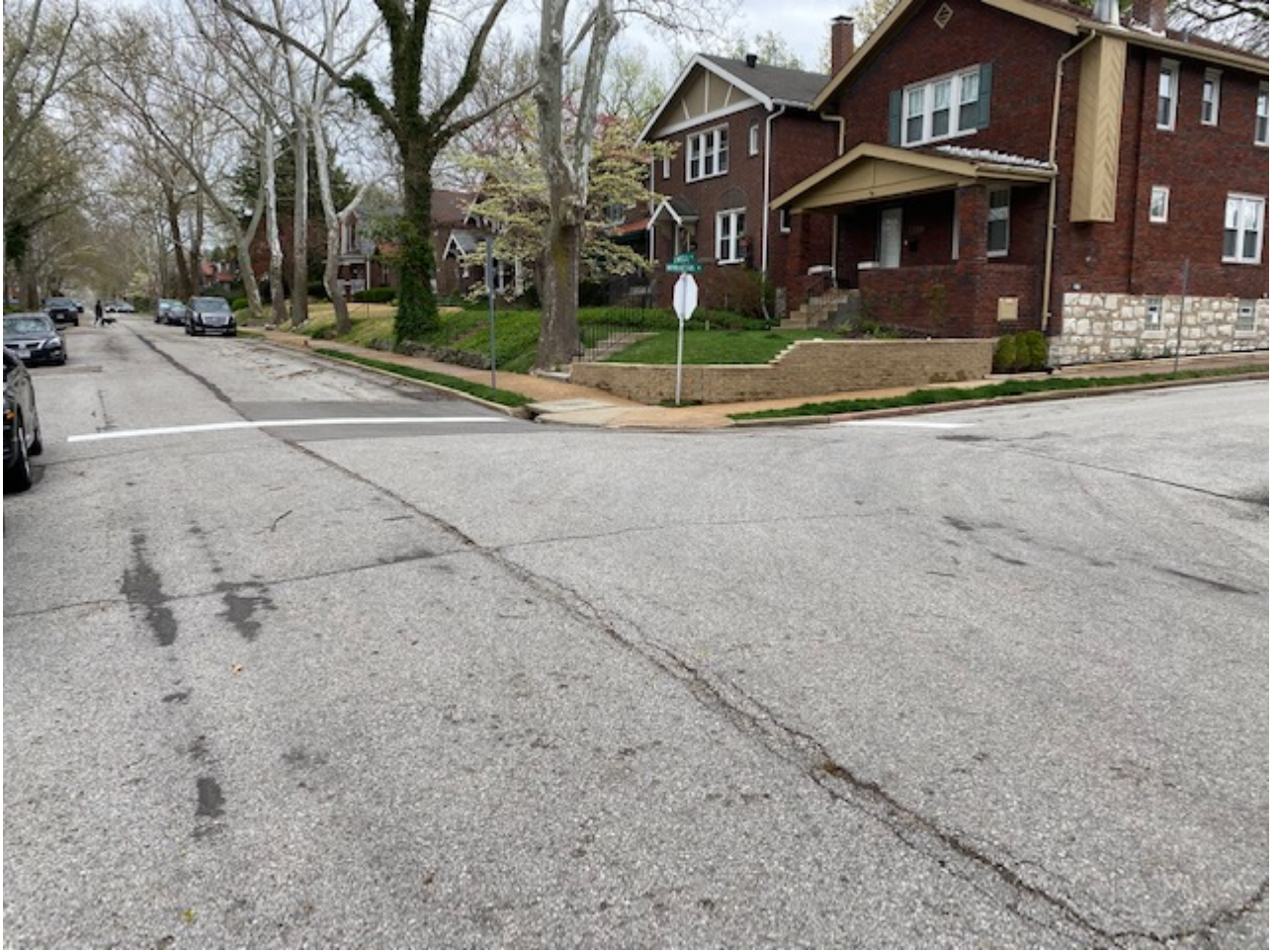
Looking southeast at Lindell (east-west) at Manhattan (north-south) intersection – newly striped stop bars
