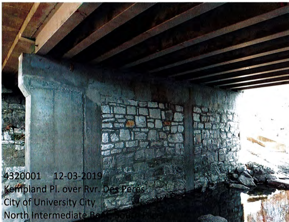
4320001 12-03-2019 Kempland Pl. over Rvr. Des Peres City of University City Fifth Girder From West at North Abutment, Pack Rust
