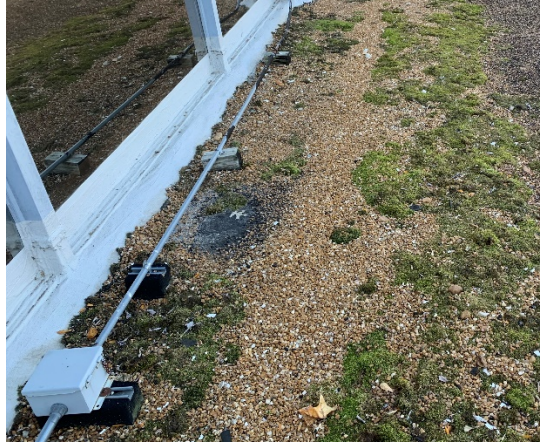
(Existing Clerestory Sill at Assembly area)
