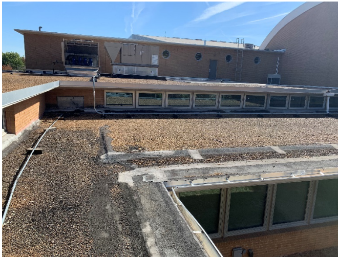
(Existing Roof and Clerestory Windows at Courtyard)
