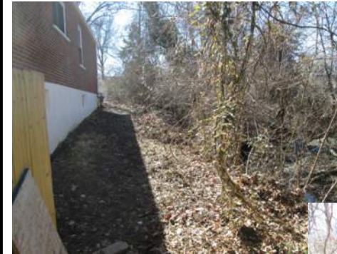
The 13-foot high eroding bank at 7591 Amherst is 9 feet from the home (measured from the top of bank).
