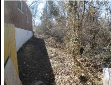
The 13-foot high eroding bank at 7591 Amherst is 9 feet from the home (measured from the top of bank).
