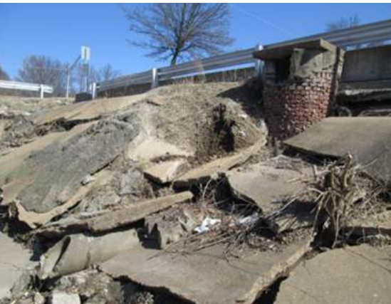
Exposed foundation of the adjacent parking lot.
