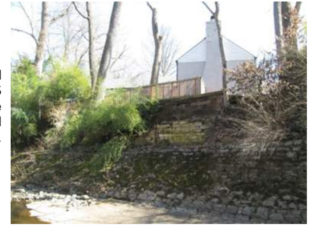
Wood tie wall and WPA block wall. 7425 Shaftesbury Ave is the house behind the wall in the photo.
