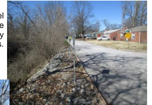
Over-steepened channel banks, and the remains of riprap placed by MSD that has since eroded and slid off the bank.
