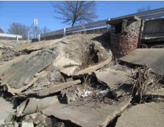
Exposed foundation of the adjacent parking lot.
