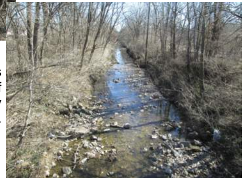
Over-steepened channel banks, and the remains of riprap placed by MSD that has since eroded and slid off the bank.
