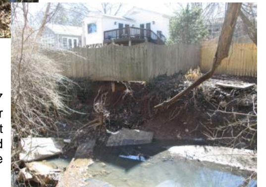
The 13-foot high eroding bank at 7591 Amherst is 9 feet from the home (measured from the top of bank).
