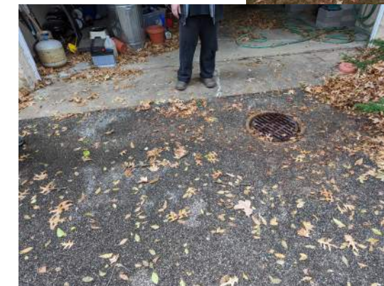
Looking at the ground in front of the driveway at 8436 Old Bonhomme Rd.
