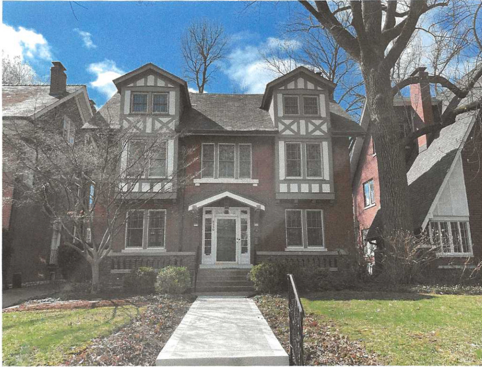
6350 Pershing Avenue North facing roof
