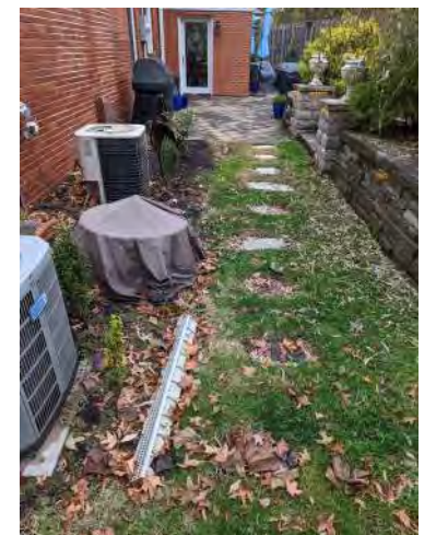
Looking east along the back of 7924 Lafon Pl. A yard drain was installed in an attempt to reduce ponding near the house.
