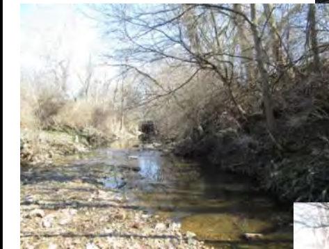
On the right descending bank are the eroding bank, collapsing fence, and sliding riprap.
