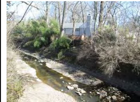
Wood tie wall and WPA block wall, looking downstream.
