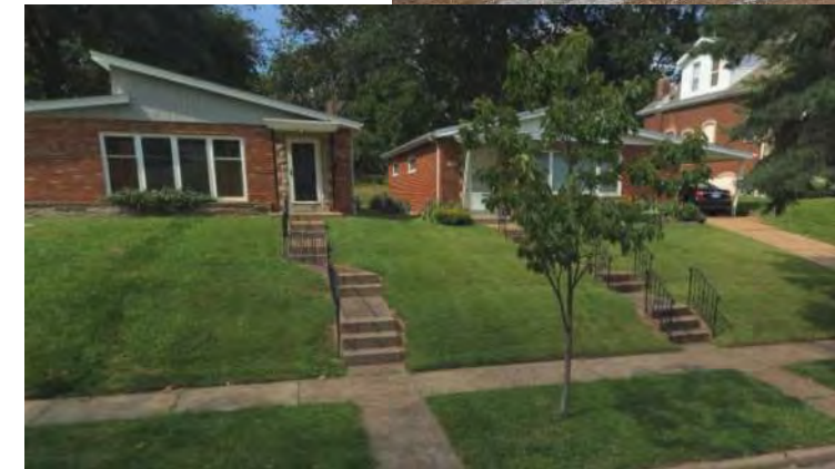
Looking north between #7423 (on the left) and #7419 (on the right). The space between houses may convey some of the runoff from the backyards, but the grading and available space is insufficient.
