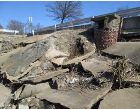
Exposed foundation of the adjacent parking lot.
