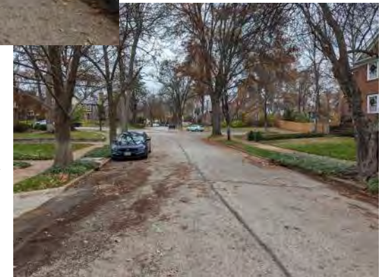
Looking north towards the northern two inlets on W Point Ct. Both are grated inlets with side intakes.
