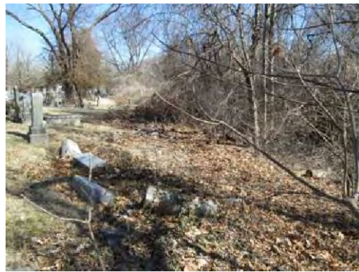
Gravestones at the B'Nai Amoona cemetery along the top of the creek bank have been damaged possibly as a result of bank erosion.
