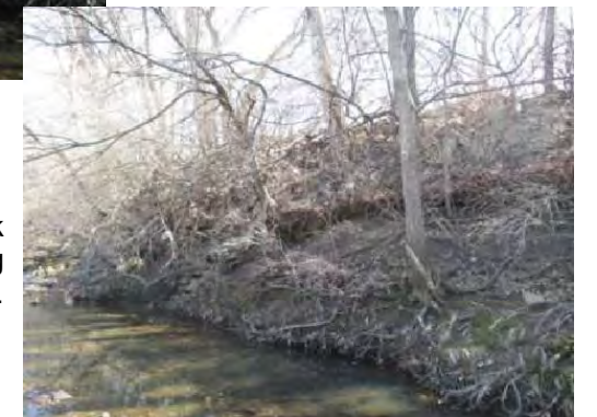
On the right descending bank are the eroding bank, collapsing fence, and sliding riprap.
