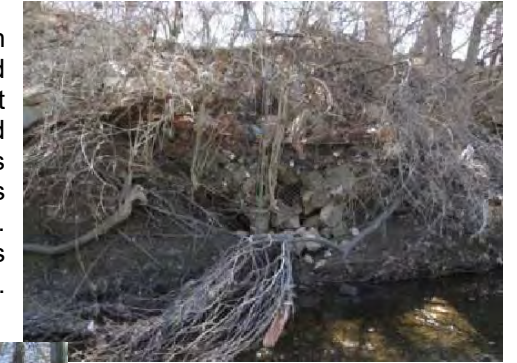
On the right descending bank are the eroding bank, collapsing fence, and sliding riprap.
