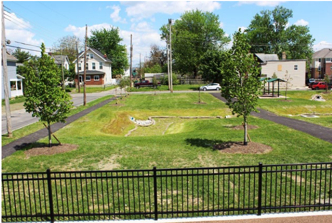
Vacant lot utilized for a stormwater management
