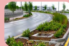
A roadway median using LID
