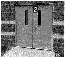
**408.5.6 Exterior access to rooms.** Doors that provide access directly into a room shall be marked with the room number or descriptive name per Section 408.4.1 directly below the exterior door identification number.
