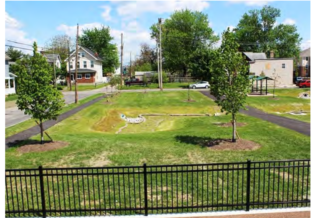
Vacant lot repurposed for stormwater management
