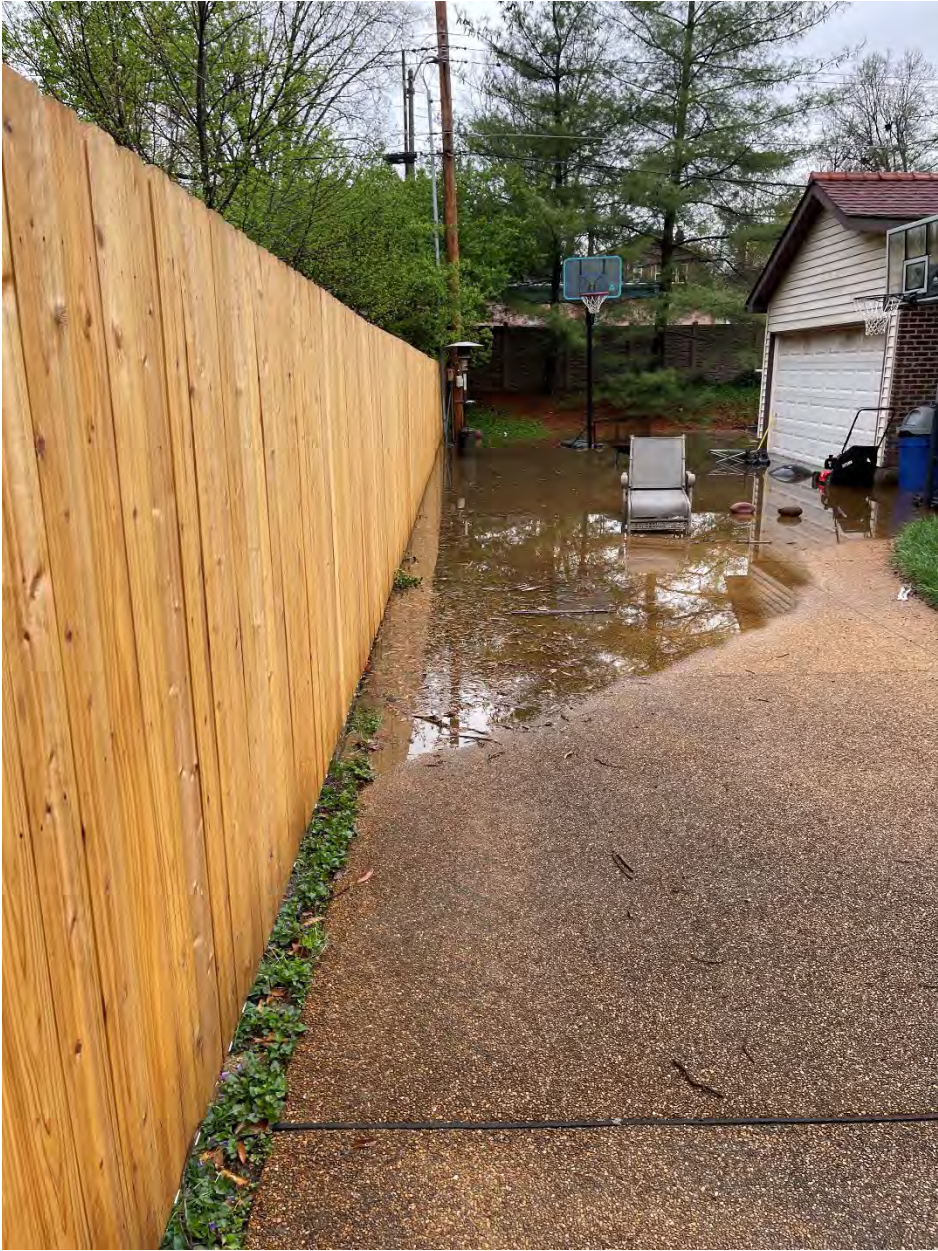
Exhibit C – Flooding Event at 7045 Westmoreland
