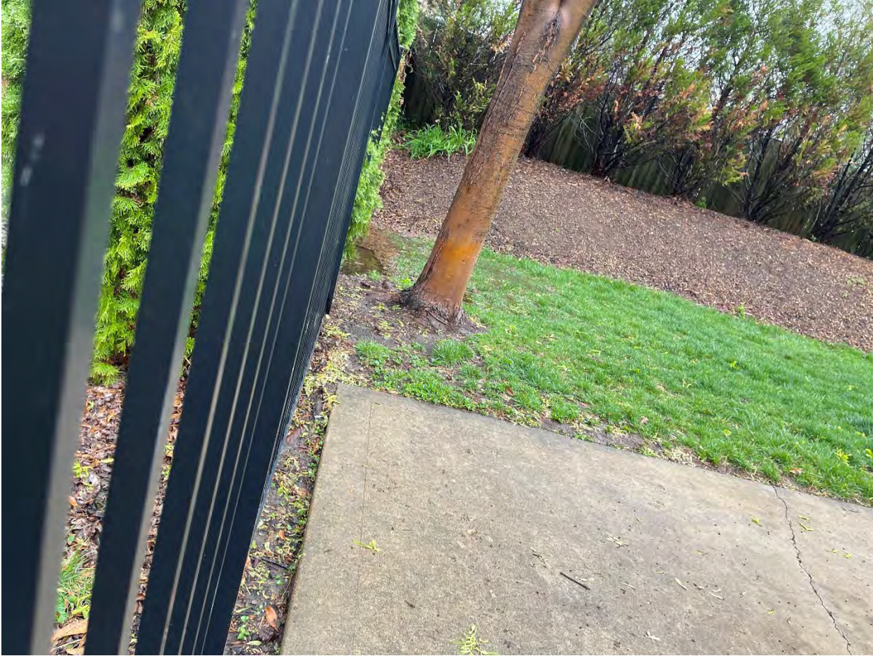
Exhibit D – Channel dammed up along the property line between 7045 and 7039 Westmoreland
