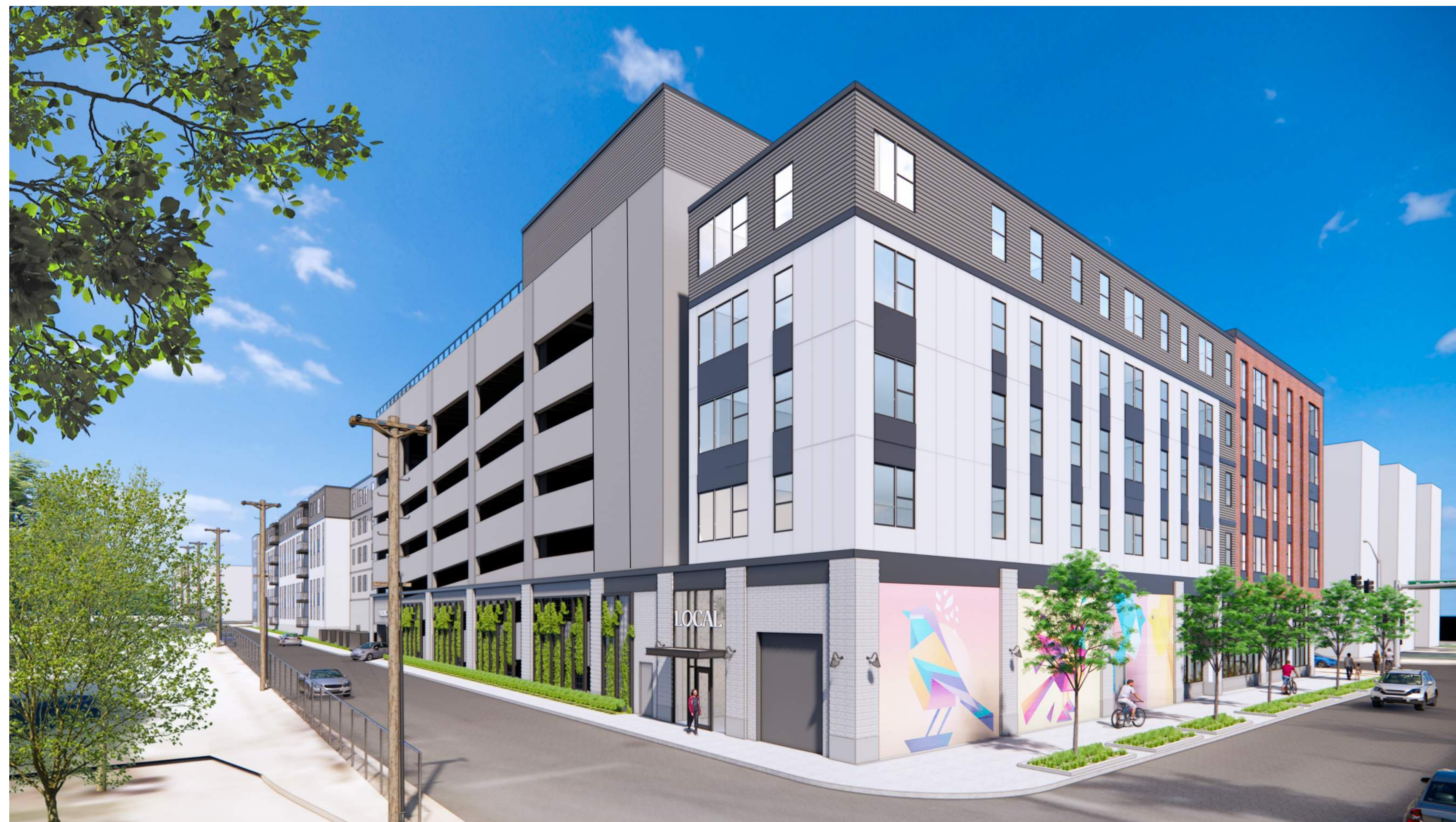
LELAND AVE & S LOOP ST
