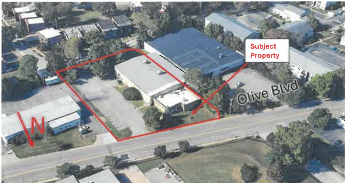
Figure 1. Aerial view of existing property.
