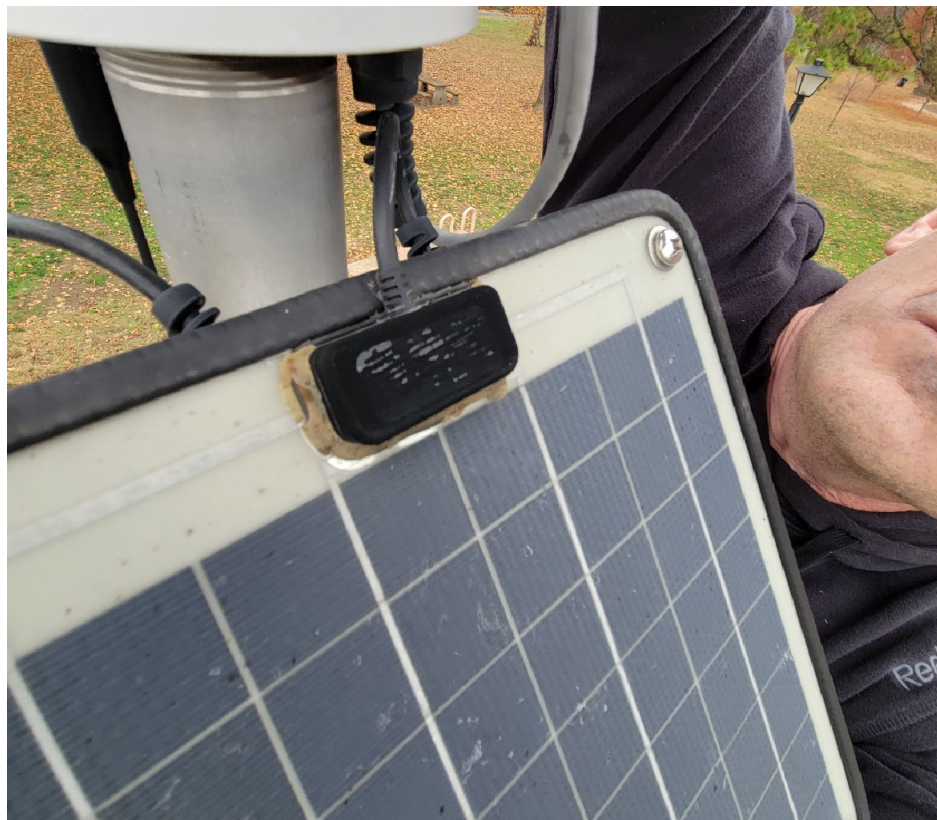
Figure 10 – Solar Panel – Silicone Detail
