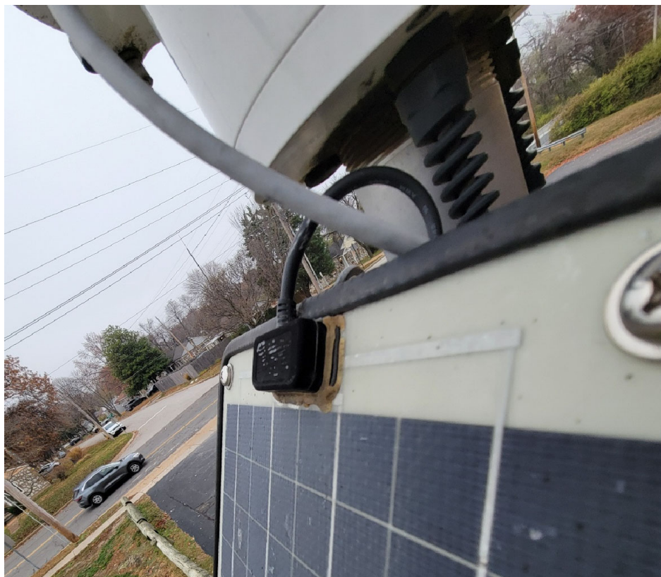
Figure 8 – Solar Panel – Silicone Detail
