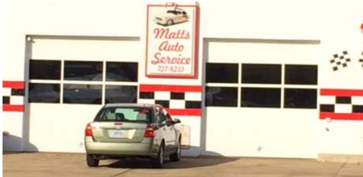
7901 Olive – New Garage Doors
